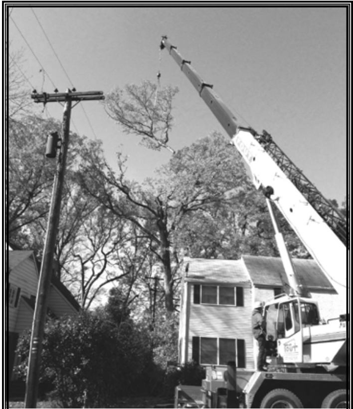
BRANCHING OUT: Using a crane, Dominion tree trimming crews are able to safely remove tree branches around elevated neighborhood power lines.
